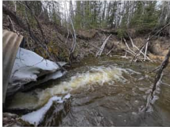
EXISTING CULVERT OUTLET.
