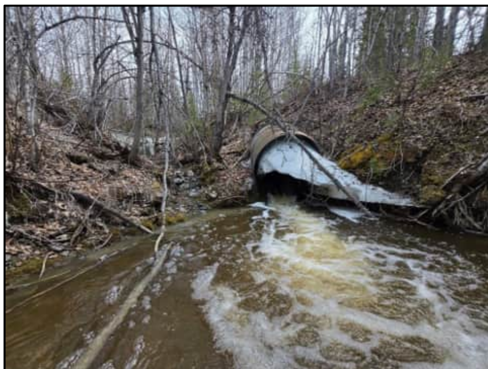
Figure 11. Outlet (looking upstream)
