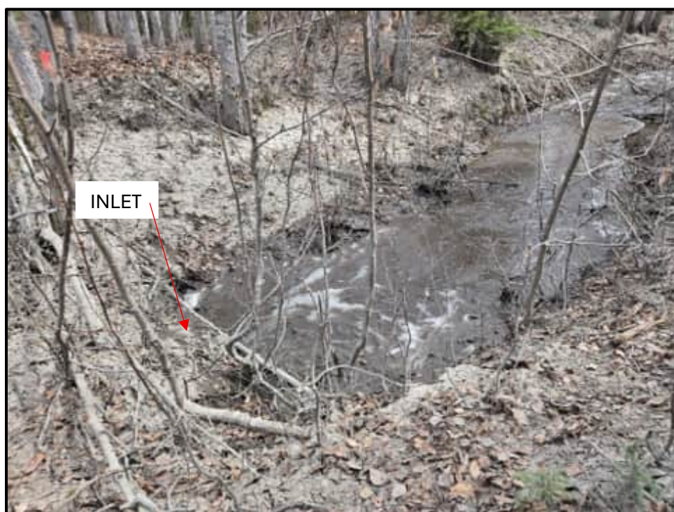
Figure 10. Inlet and upstream reach (looking upstream)
