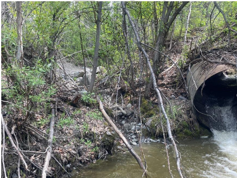
View: Looking upstream at washout next to outlet.
