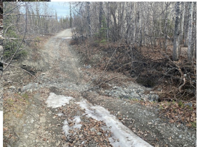
Figure 2: Photos of the ATV crossing to be decommissioned and the perched culvert at Little Tonsina Tributary
