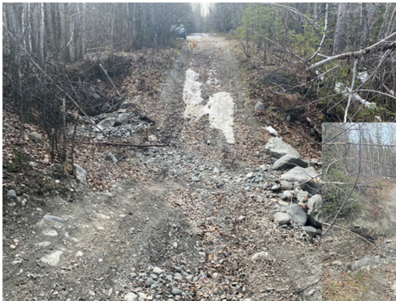
Pictures of the trail looking both ways through the crossing. Note the significant wash-out and steep road gradient.
