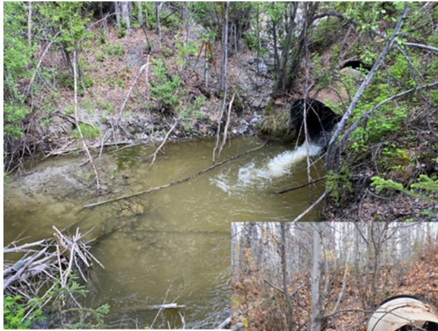
Pictures of the culvert outlet and associated scour pool.
