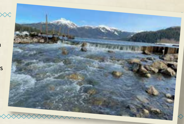
(Below) Looking upstream at the old Eyak Lake Weir that is currently in the planning stage for replacement. Photo by Euan-Angus MacLeod
