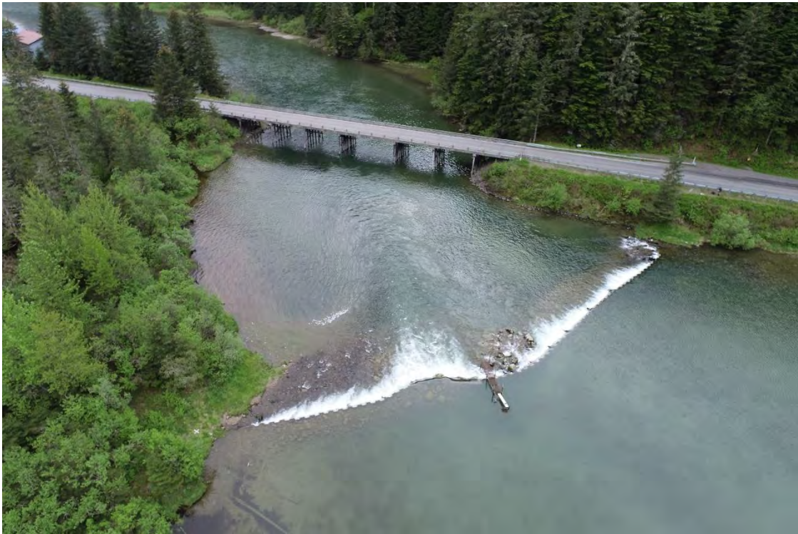
Figure 1: Eyak Lake Weir and Copper River Highway Bridge
