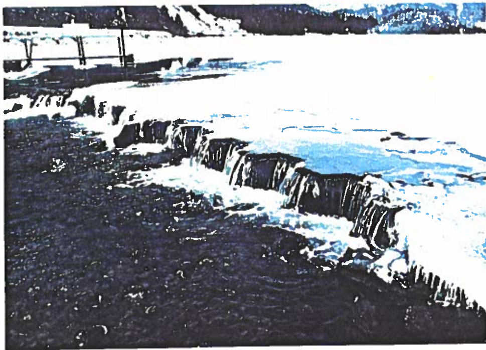
Photo No. 2 Westerly View of Dam Boatway - Upper Left
