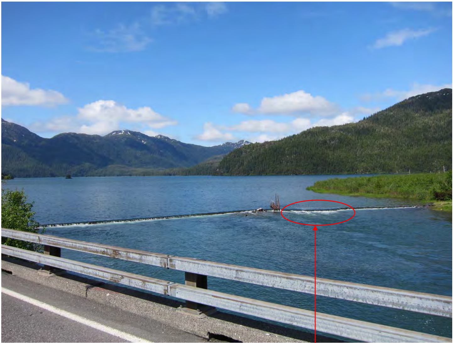
Boat Slot and Partially Failed Section
