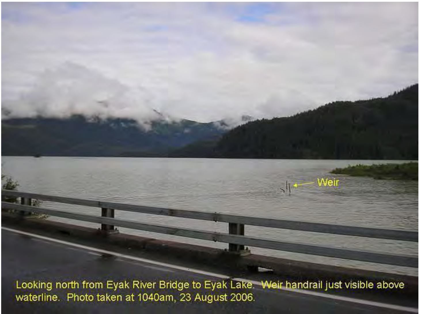
Weir Submerged at Stage 24.52' Unknown Datum (Photo Courtesy of National Weather Service)
