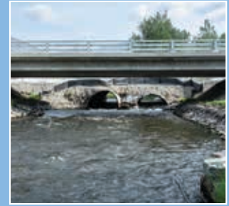
Vegetation starts to regrow at the recently completed Little Tonsina Bridge.
