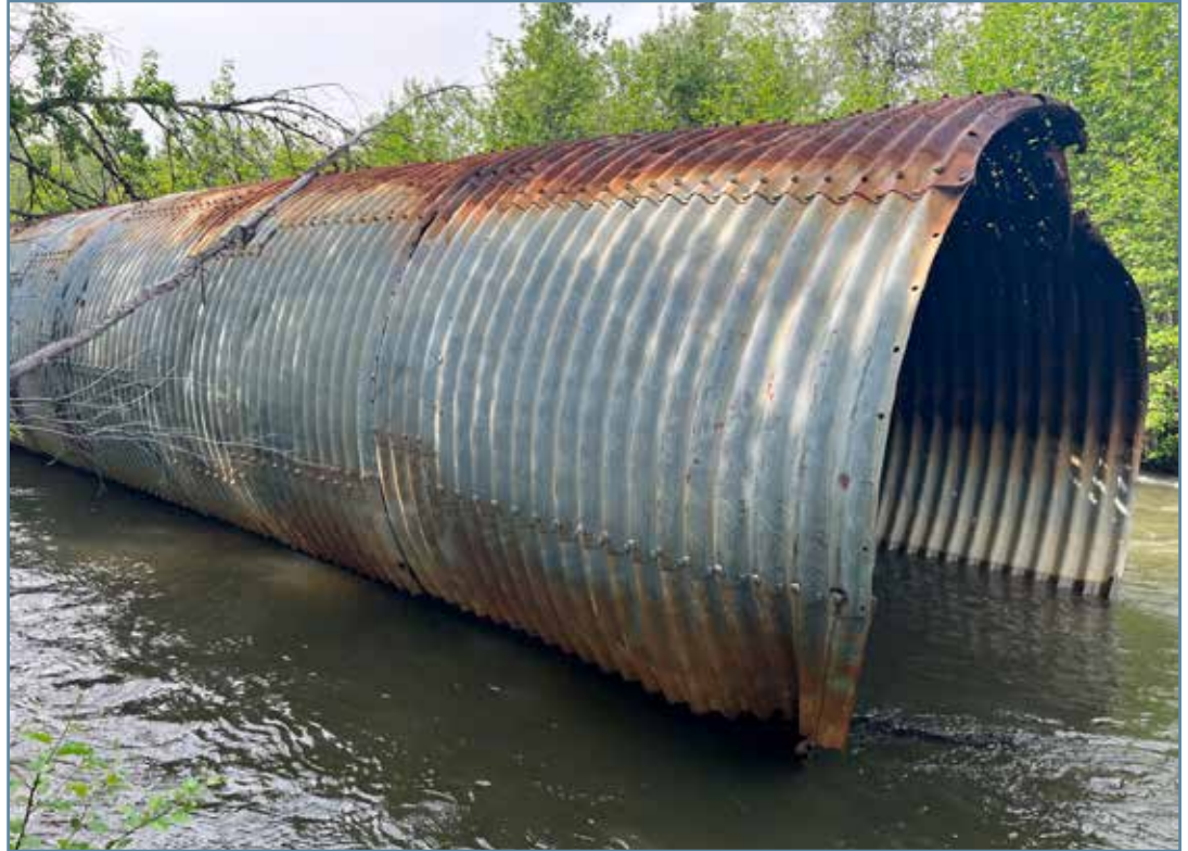
An undersized culvert that was carried downstream by the 2006 flood on the Little Tonsina River. Picture from K. Liebich, USFWS.
