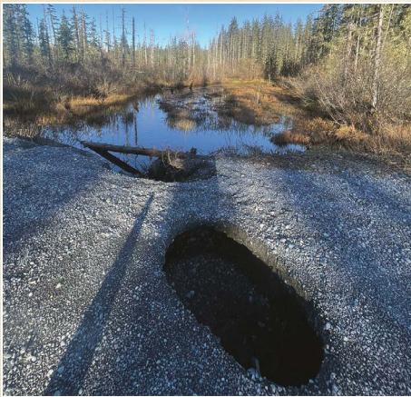
Sinkholes on the Copper River Highway were caused by high flows being constricted by small culverts, forcing water through the road bed and causing material around the culverts to erode.
