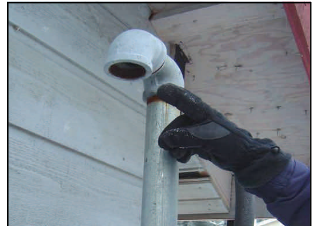
Check the tank vent for any obstructions like snow, ice, insects or spiders.
