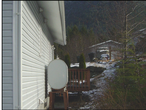
Check for ice, snow or tree limbs that can fall on your tank or fuel lines. Photo shows a tank at risk of ice and snow falling on it during the winter.
