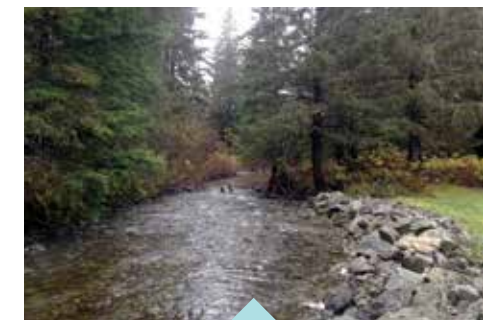
Rip rap installed by homeowners to armor stream bank.
