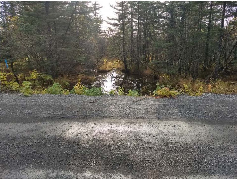
COP 45 downstream side looking downstream from road surface
