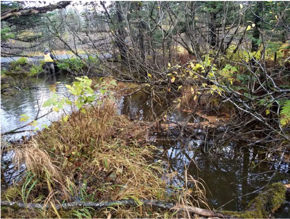
COP 45 downstream side looking upstream to culvert
