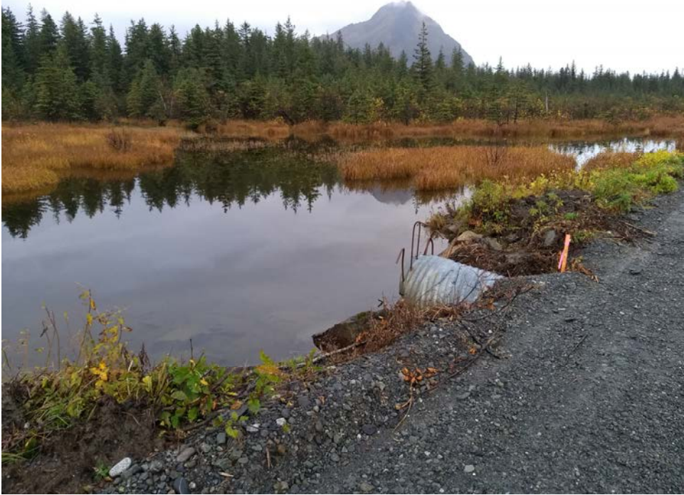
COP 43 upstream side
