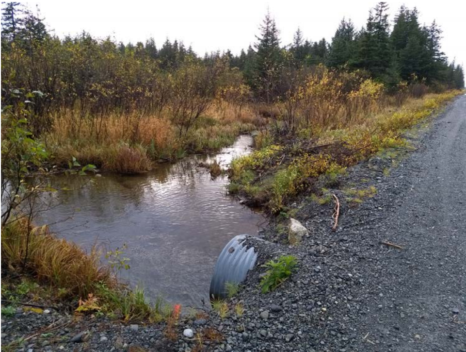
COP 43 downstream side
