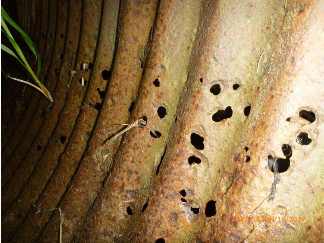
CRH mile 21.4 Pipeline Trail Creek Inlet
