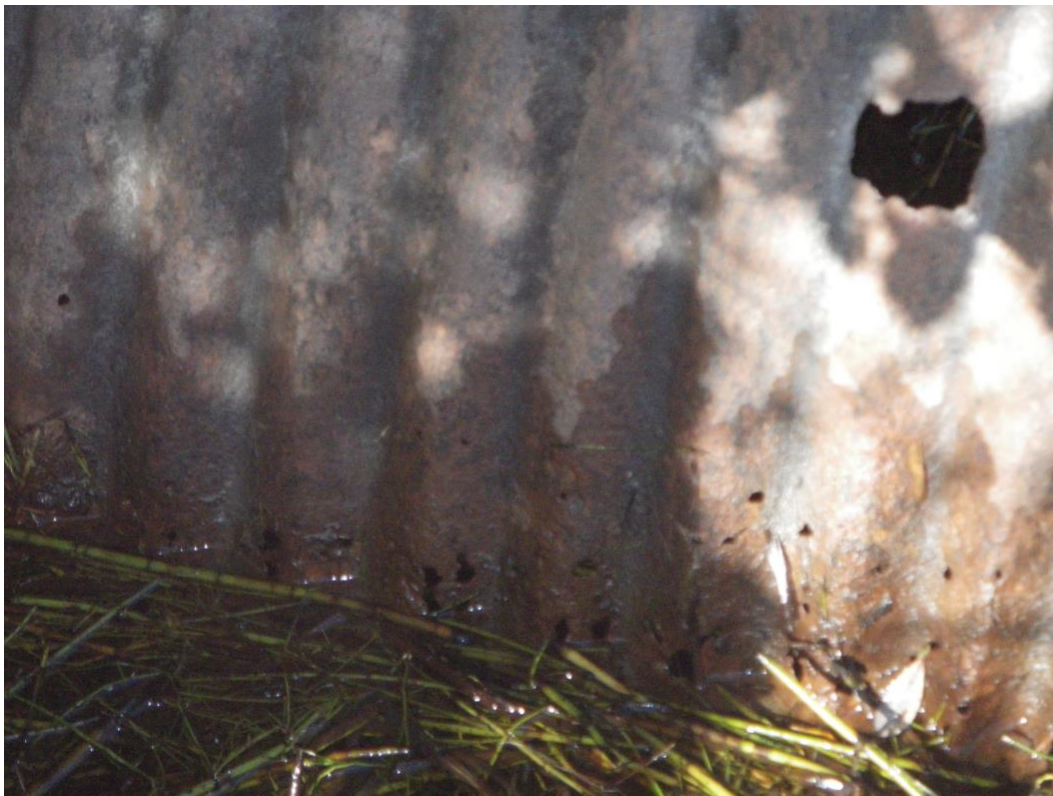
CRH Mile 19.7 - Rusted Inlet
