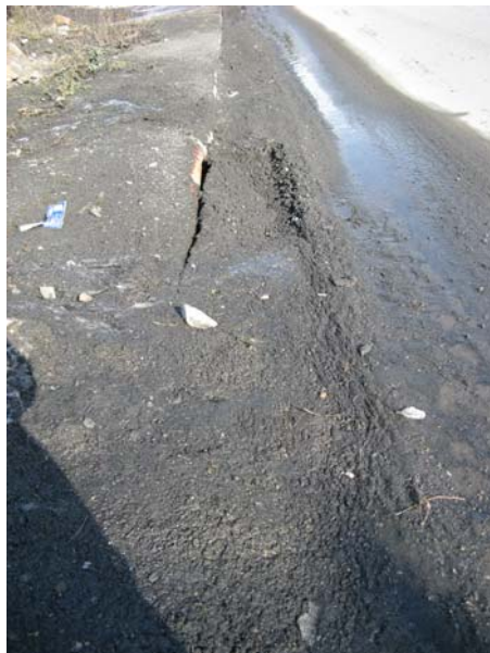
Photo No. 8 Storm drain, sediment-inundated in spring
