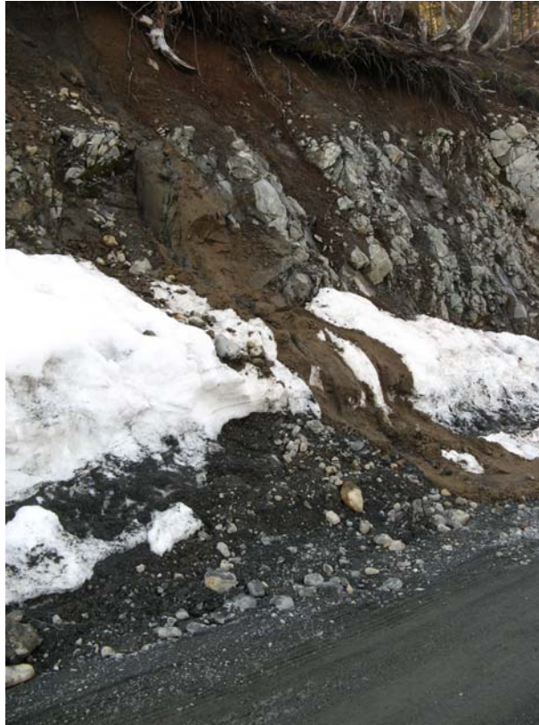
Photo No. 5 Construction site mud flow from a cut bank, Eyak Lake area
