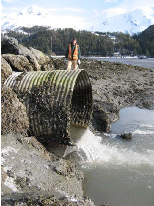
Photo No. 7 Main Orca Inlet outfall, 6-foot culvert
