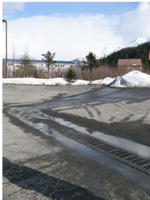
Photo No. 2 Hospital parking lot sediment-filled trench drain
