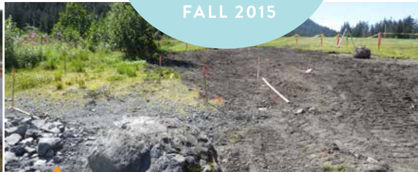
AFTER: RE-GRADING OF SNOW STORAGE SITE CREATES A DRAINAGE SWALE TO ALLOW FOR BIO-FILTRATION AND SEDIMENT TRAP CAPTURE OF POLLUTANTS BEFORE SNOW MELT REACHES ODIAK POND.
