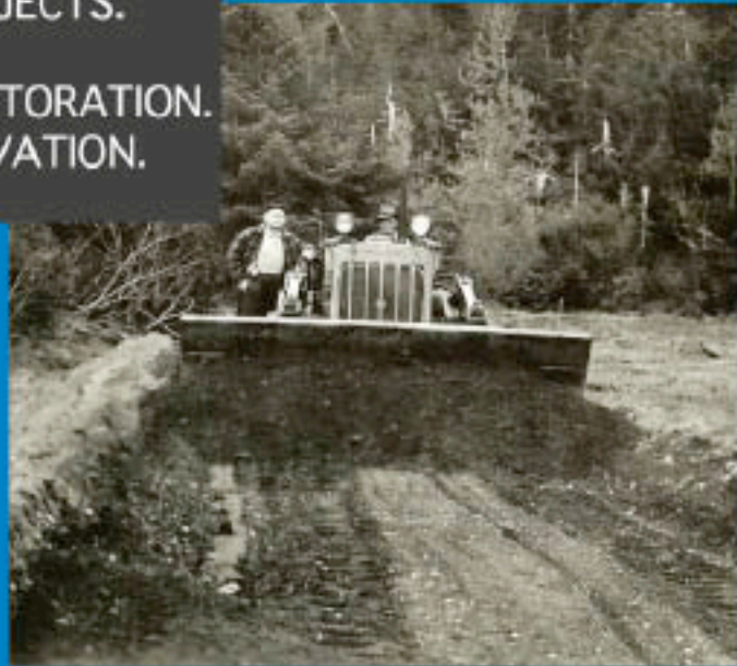
Picture courtesy of Cordova Historical Society. Construction around Eyak Lake.
